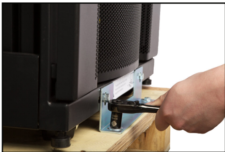
Removing the Bolts
